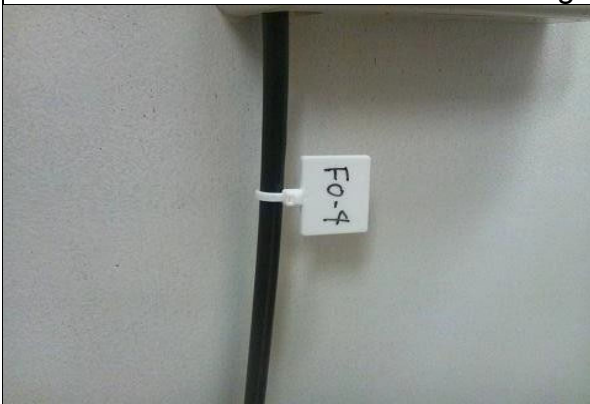
Labeling fiber cable on cable ladder/wall (Not recommend).
