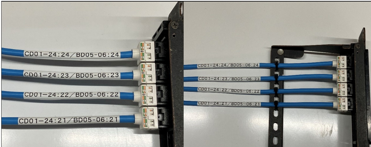
Labeling xTP cable end.
